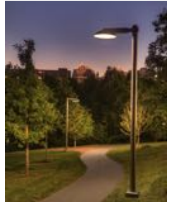
Appropriate parking lot lighting will meet the night sky lighting standards.
